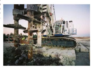
The soils were mixed in situ with predetermined quantities of binder, a blend of Slag and Portland cement. The grout was injected at the bottom of the drilling rods at different rates of pressure and flows to address the peculiar properties of each soil layer.
